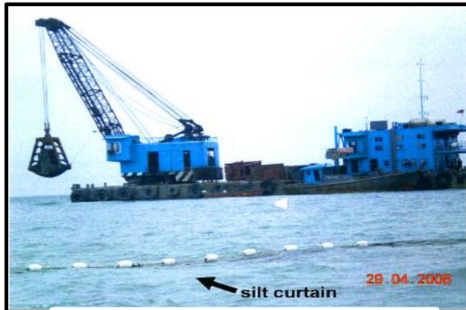
Silt curtain was erected and maintained properly
