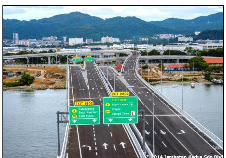
Internally lit signages should be used where elimination of the external light sources and associated grating and support is beneficial.
